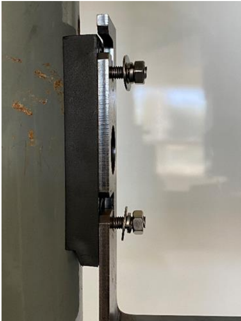
Figure 1: Slotted bracket with temp fixing kit
